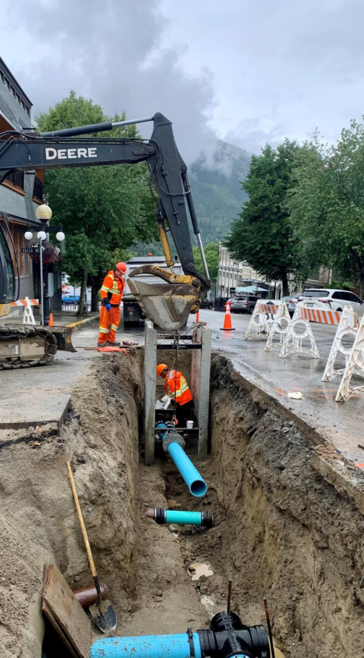
Photo: Staff working on the Baker St main replacement
