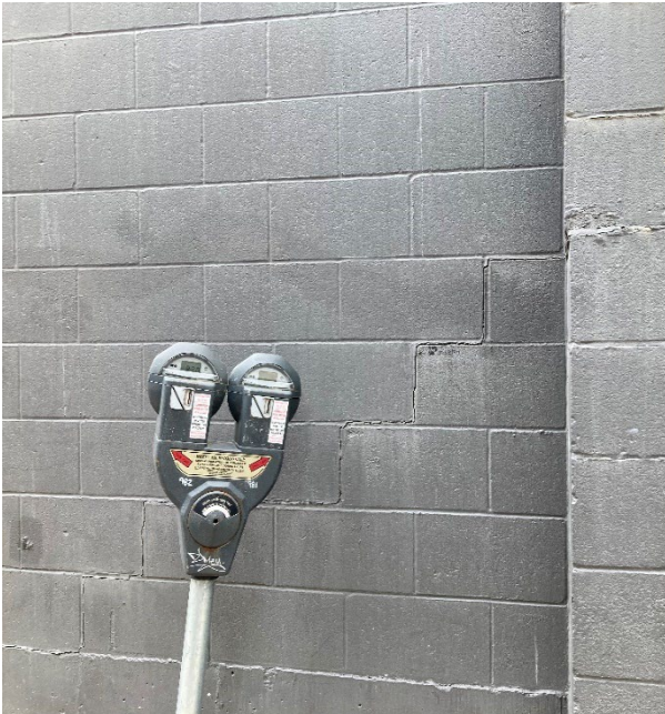
Photograph 1: Cracking of Mortar Between Masonry Blocks on East Curling Rink Wall – Facing West
