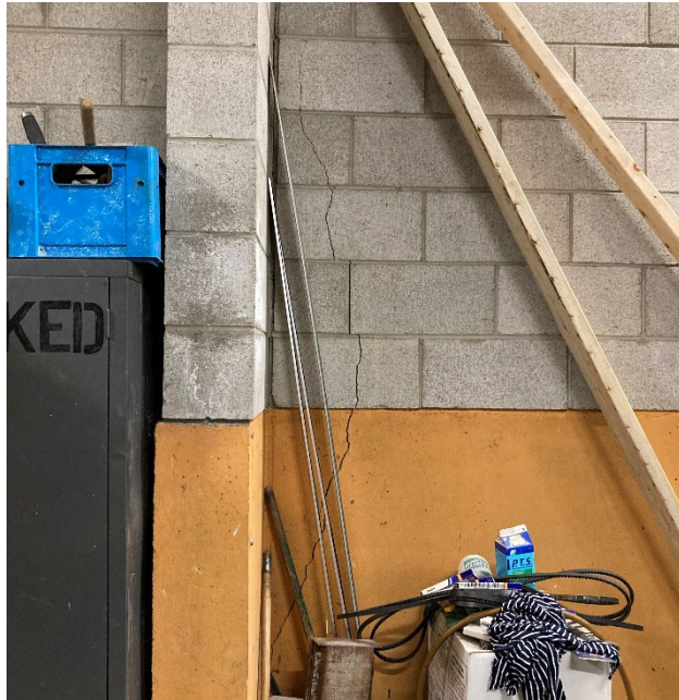
Photograph 2: Cracking Inside Refrigeration Equipment Room (South Wall) – Facing South
