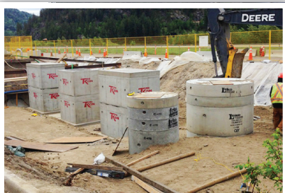
Photo above: The grit chamber actually sits below all these risers.
