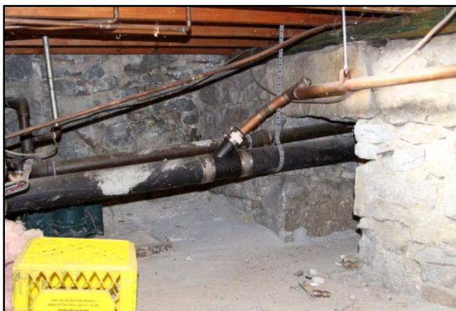
Photograph 8 – Perimeter and intermediate, stone foundation walls with the lower level floor overhead.
