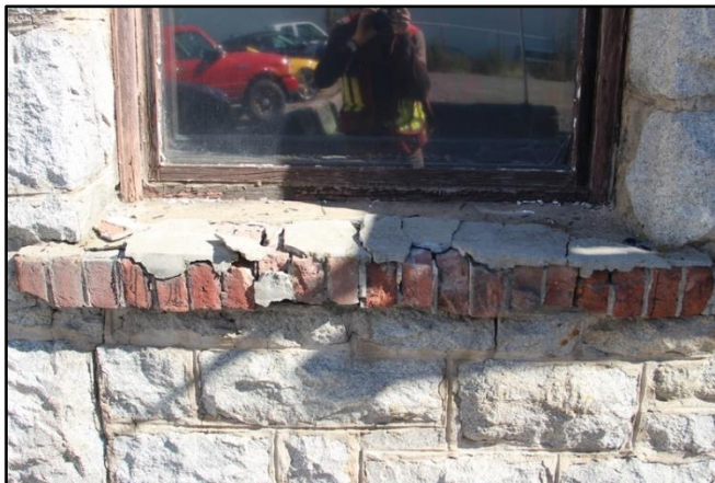
Photograph 6 – Granite block wall beneath a clay brick window sill with failed parging.
