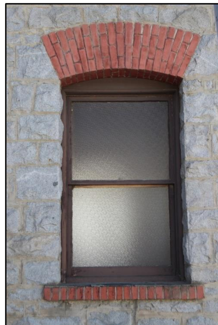
Photograph 7 – A lower level, hung sash window with opaque glass.
