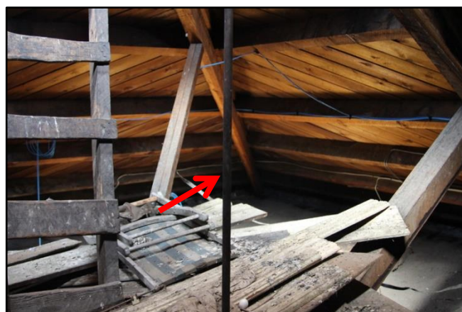
Photograph 5 – The heavy timber roof structure with horizontal purlins and shiplap planks. Note the central steel tie rod.
