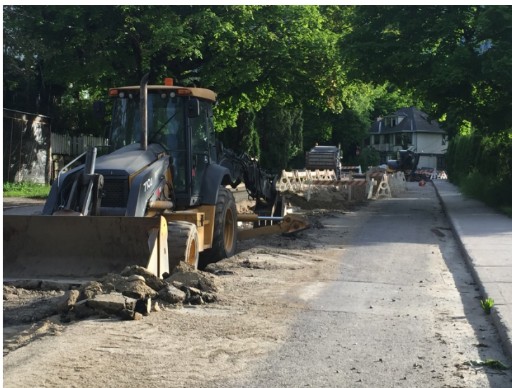
Water Main work taking place on Hall Mines Road.
