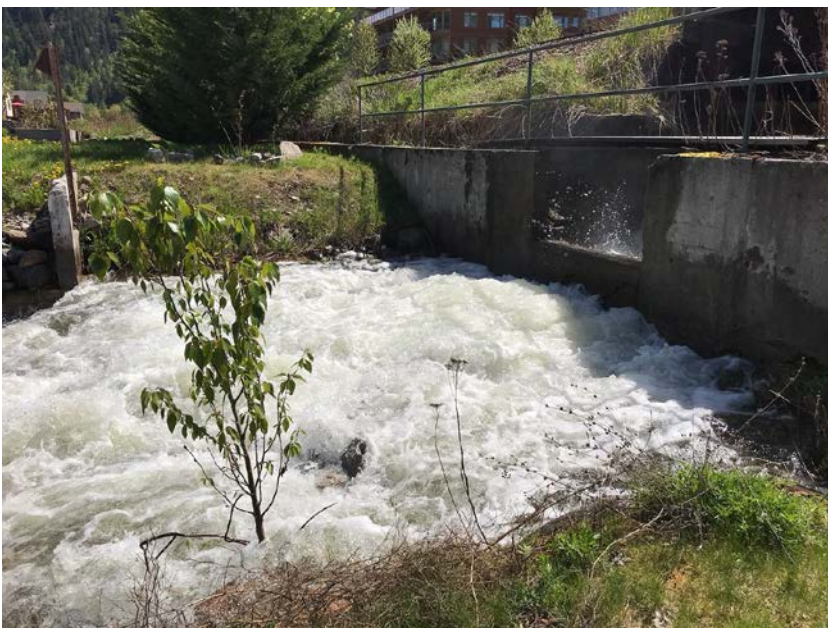
Anderson Creek in Fairview
